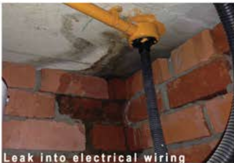
Leak into electrical wiring
