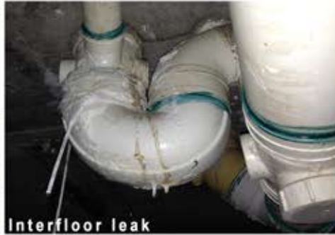
Interfloor leak
