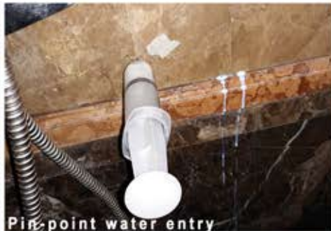
Pin-point water entry
