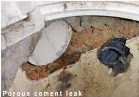
Leak into electrical wiring
