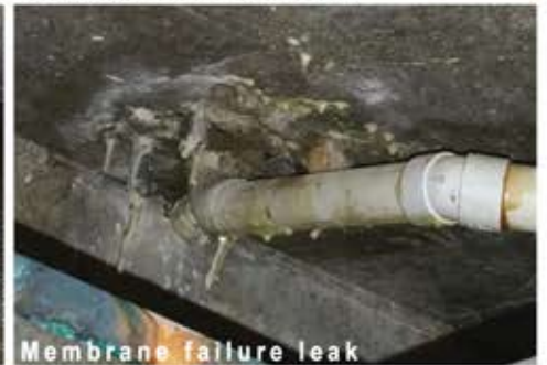
Tracing leak flow path
